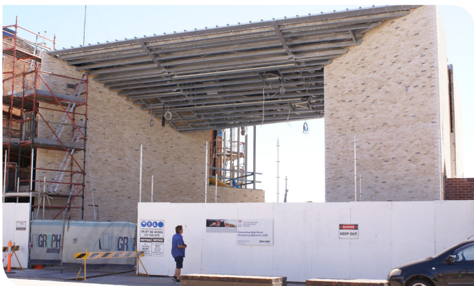
View from High Street side
